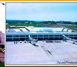
DAVAO AIRPORT OPERATIONS, MAINTENANCE & DEVELOPMENT PROJECT
