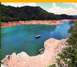
BULACAN BULK WATER SUPPLY PROJECT
